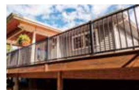
Antiseptic LVL installed in the wood deck
