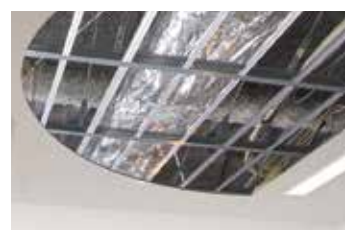
Our own anti-seismic ceiling construction technique
