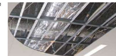
Our own anti-seismic ceiling construction technique
