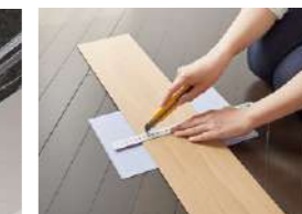
Flooring for renovation that can be easily constructed in a short construction period
