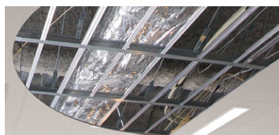
Our own anti-seismic ceiling construction technique
