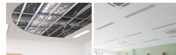
An anti-seismic ceiling construction technique
